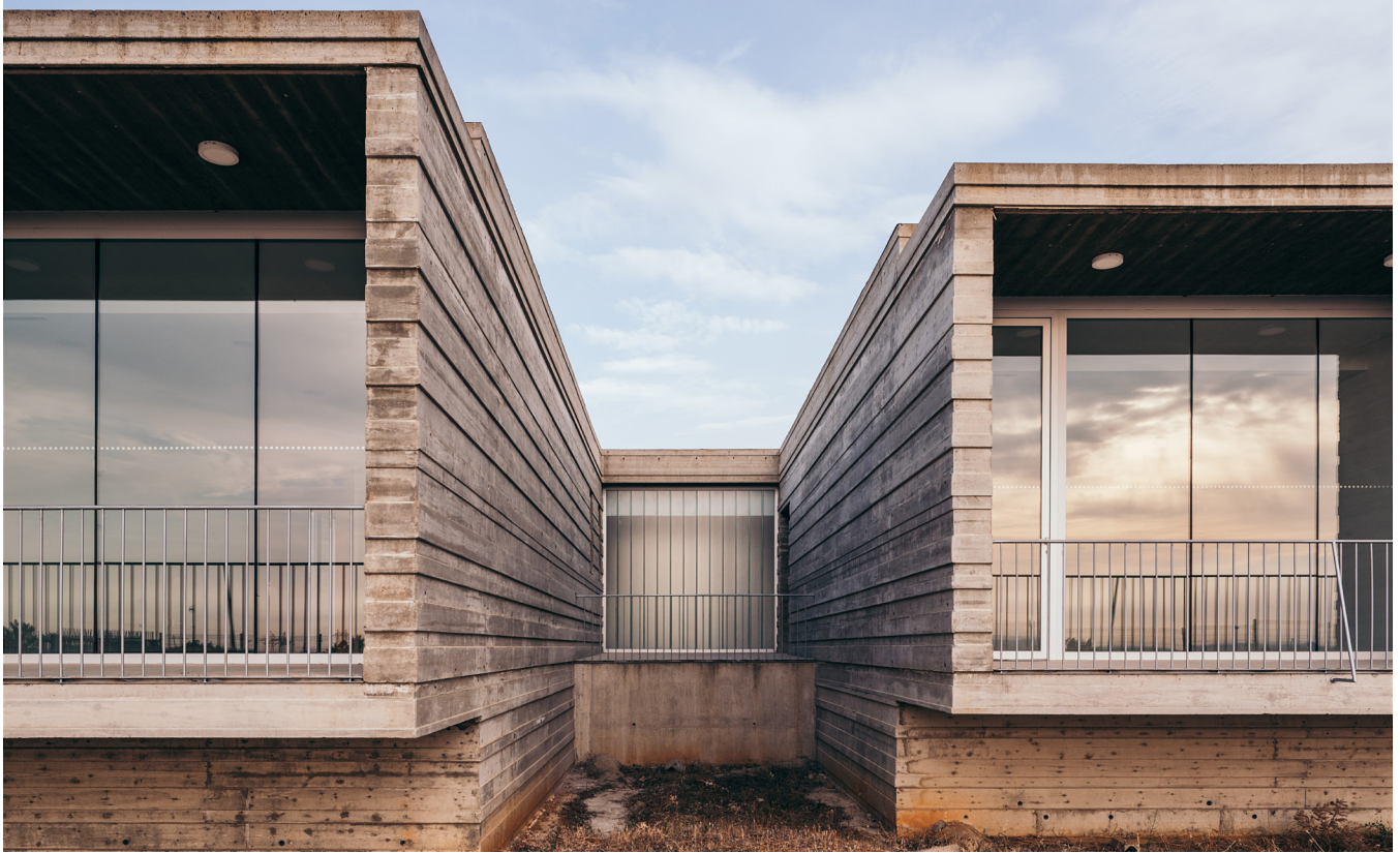
Figure 4. Detail View of the Classrooms and External Courtyard. Javier Bravo Photography.
