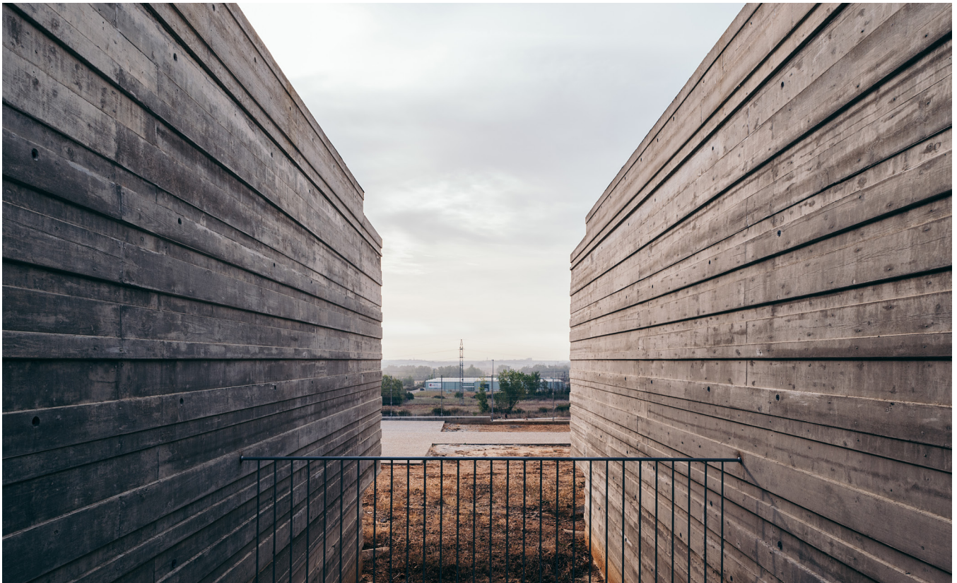
Figure 5. Detail View of the Classrooms and External Courtyard. Javier Bravo Photography.
